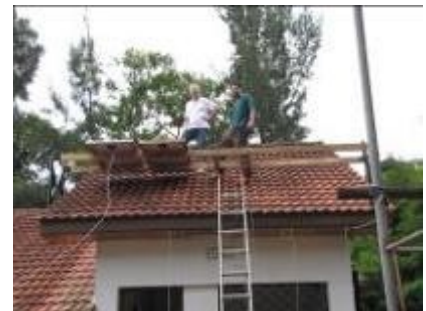
Stan and Ricky installing the solar panel support platform
